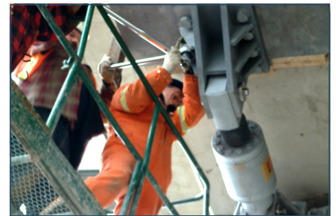
Site Installation Bolt Torquing
